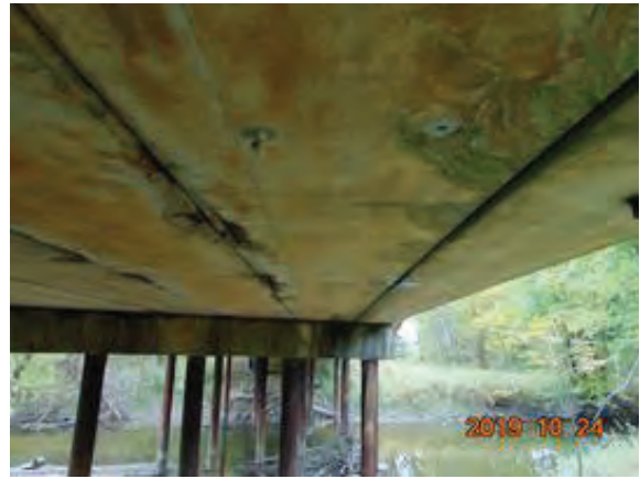
File Description Looking at Beams A3-4 - Spalls
