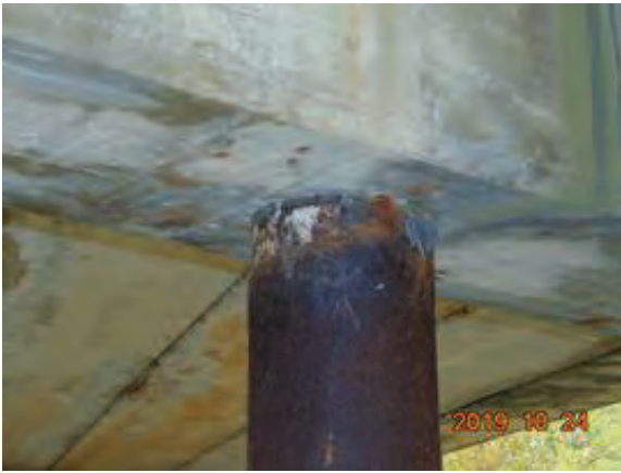
File Description Looking at Bent 2 Pile Rust Through
