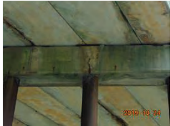
File Description Looking at Bent 4 - Spalling
