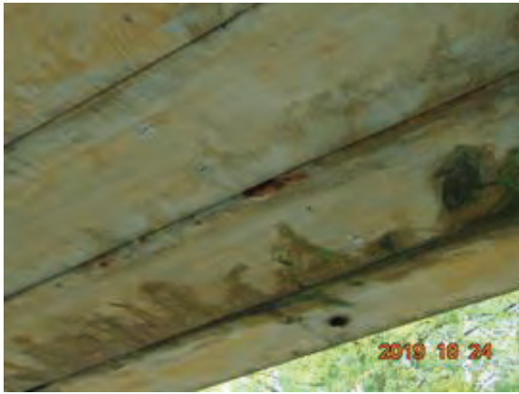
File Description Looking at Beam C2 - Spalling
