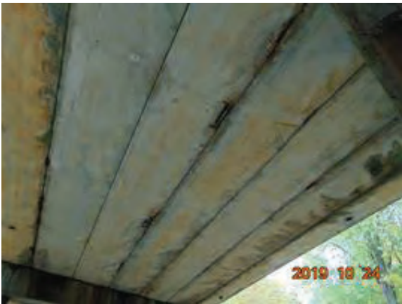
File Description Looking at Beams C4 & C5 - Spalling File Type Category
