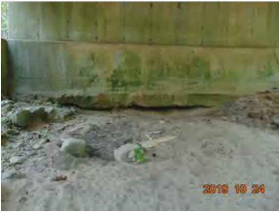
File Description End Bent 5 Deterioration due to Socur
